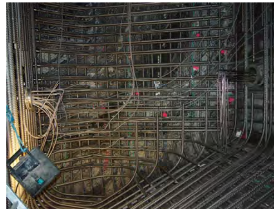
PVDF and stainless steel tubes, directing the pressure sensor cables to the cable flanges towards the filter layer (right side) and plug section 2 (left side)
