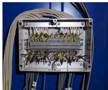
Leakage box for interrupting potential water leakage along and inside the wires
