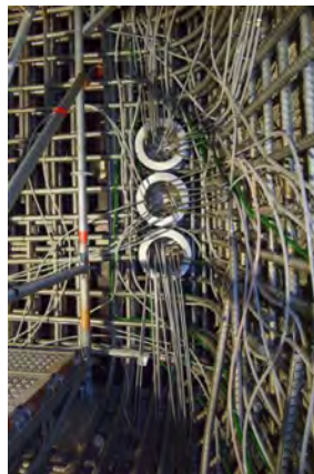
Three cable flanges, which carry in total 51 sensor wires, photographed from inside (left) and outside (right) plug section 2
