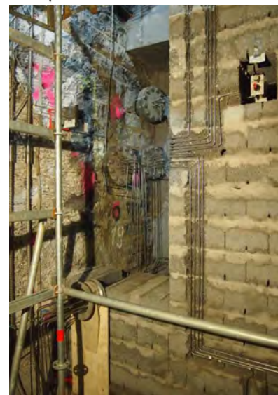
stainless steel tubes for hosting the sensor wires, mounted onto the filter layer wall
