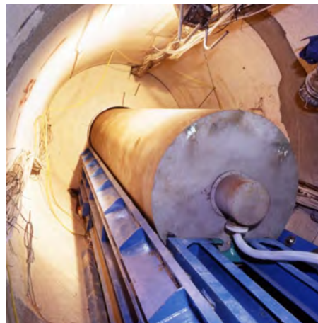
Disposal in horizontal drifts
